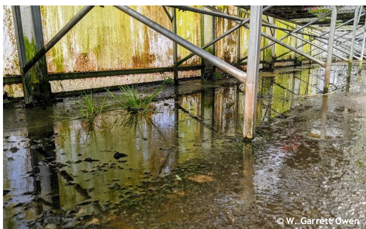
Figure 17. Floors that are wet and covered in algae are significant safety hazards to team members, increasing the likelihood of slipping risks. Photo by: W. Garrett Owen, OSU.
