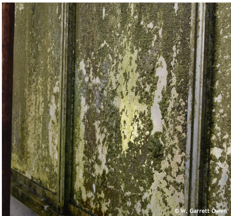
Figure 18. Example of a propagation side wall covered in algae thereby serving as an area for continued growth and reduced light transmission. Photo by: W. Garrett Owen, OSU.
