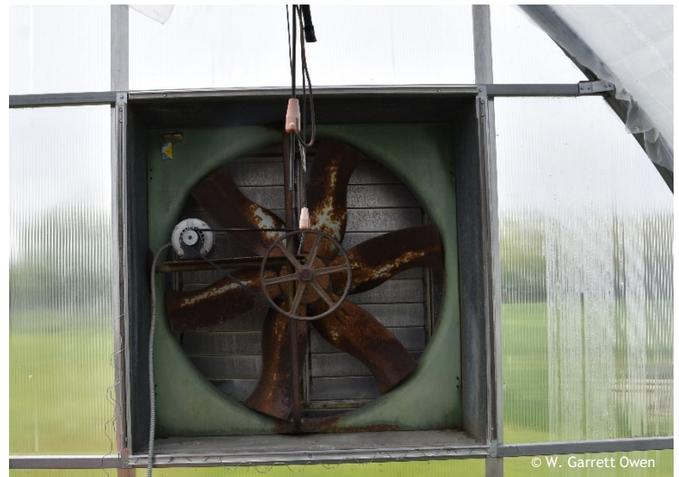
Figure 10. Installation of a new exhaust fan belt. Photo by: W. Garrett Owen, OSU.
