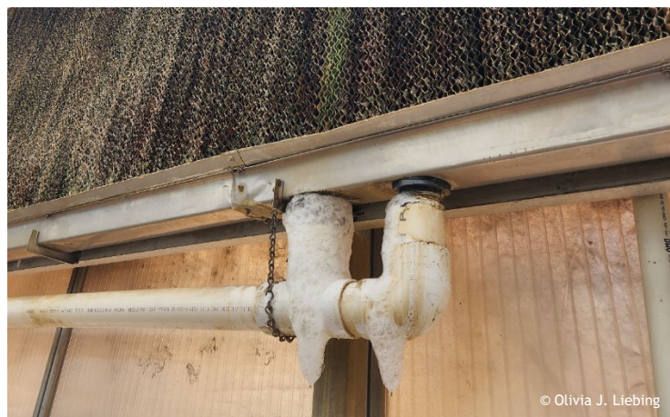
Figure 7. Water is leaking out of the return pipe from this pad-and-fan system, not only reducing efficiency but creating a puddle below in a busy walkway. Photo by: Olivia J. Liebing, OSU.
