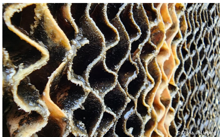
Figure 4. Algae build up on cooling pads can greatly reduce pad efficiency and life span. Photo by: Olivia J. Liebing, OSU.
