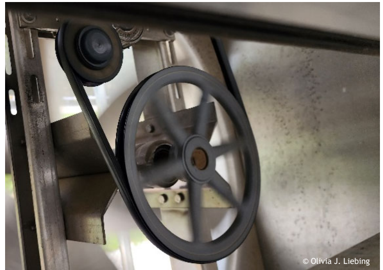
Figure 9. Over time, exhaust fan belts can become loose, cracked, or worn. Photo by: Olivia J. Liebing, OSU.
