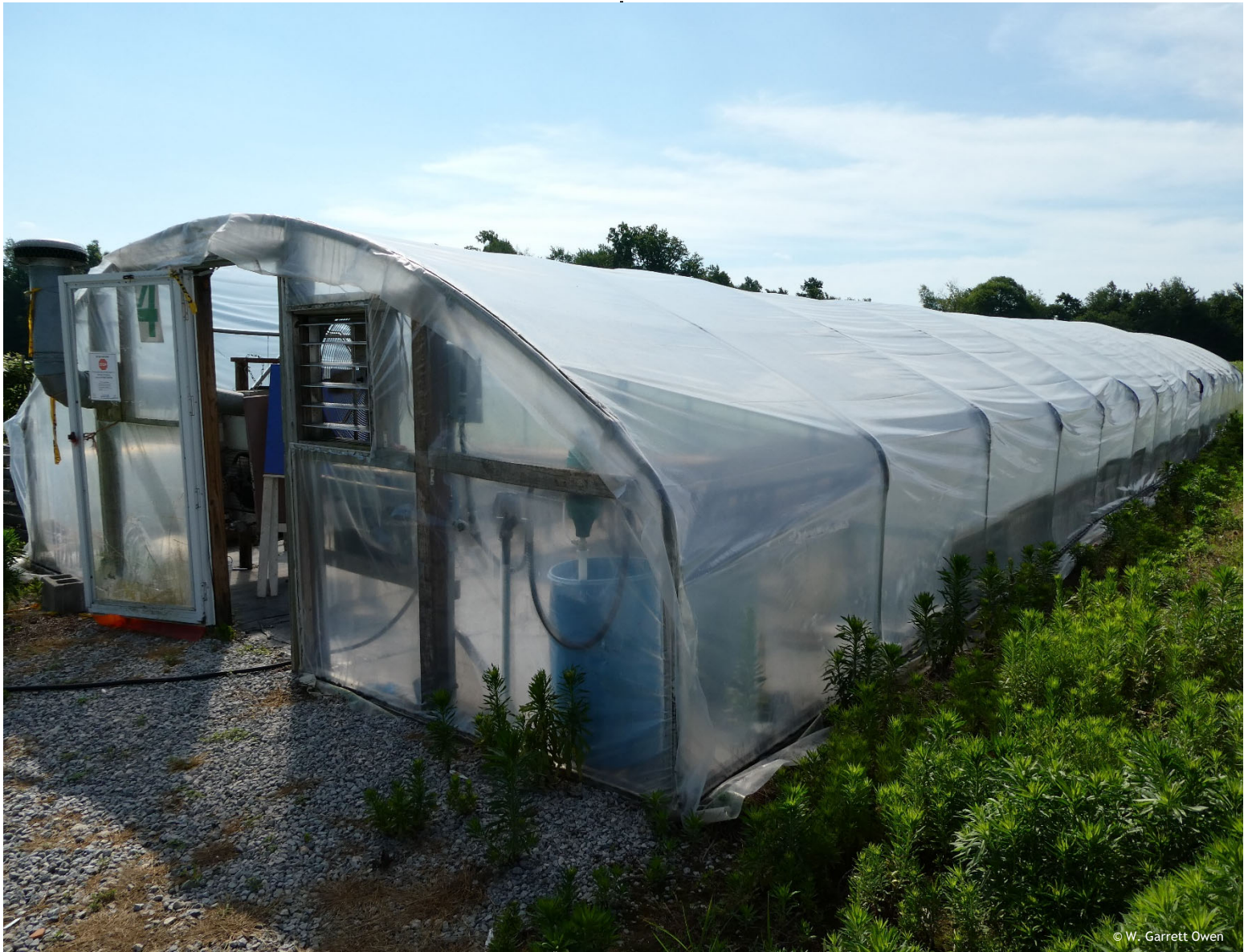
Figure 12. Leaving greenhouse door ajar significantly reduces the overall airflow across the greenhouse, diminishing the cooling capacity of the pad-and-fan system by allowing cooled air to escape or hot air to enter without passing through the pads. This action reduces the effectiveness of temperature control during the summer. Photo by: W. Garrett Owen, OSU.
