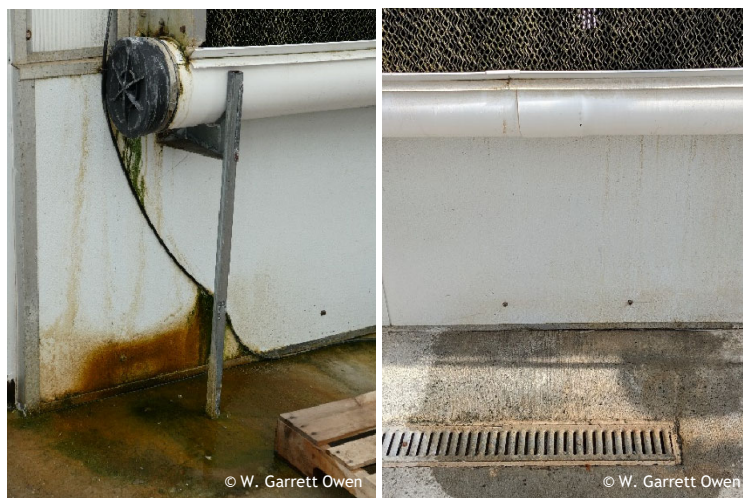
Figure 8. Leaks from cooling pads and gutters can create hazardous puddles on the greenhouse floor which pose a slip risk for employees, can damage flooring or nearby equipment, and promote algae growth. Photos by: W. Garrett Owen, OSU.
