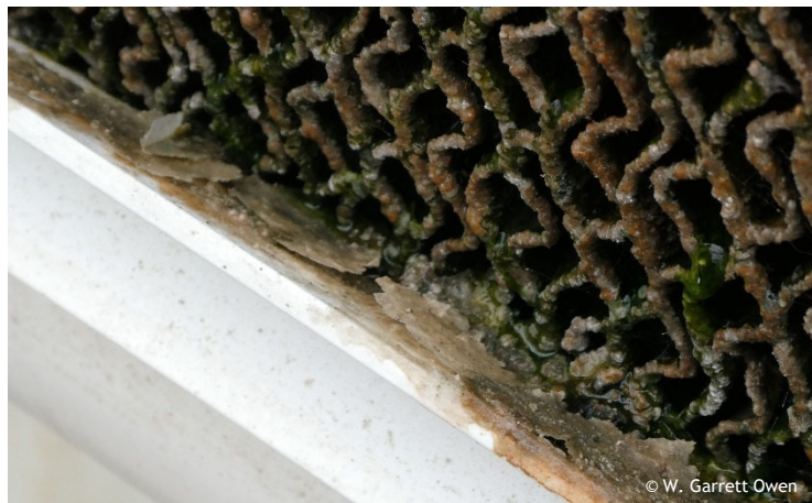
Figure 6. Mineral deposits such as salt or calcium can accumulate on the pad surface as water evaporates and leaves particulates behind thereby reducing cooling efficiency. Photo by: W. Garrett Owen, OSU.
